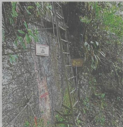
One of the 17 metal ladders on the Pinnacles route is bolted into the cliffside.
